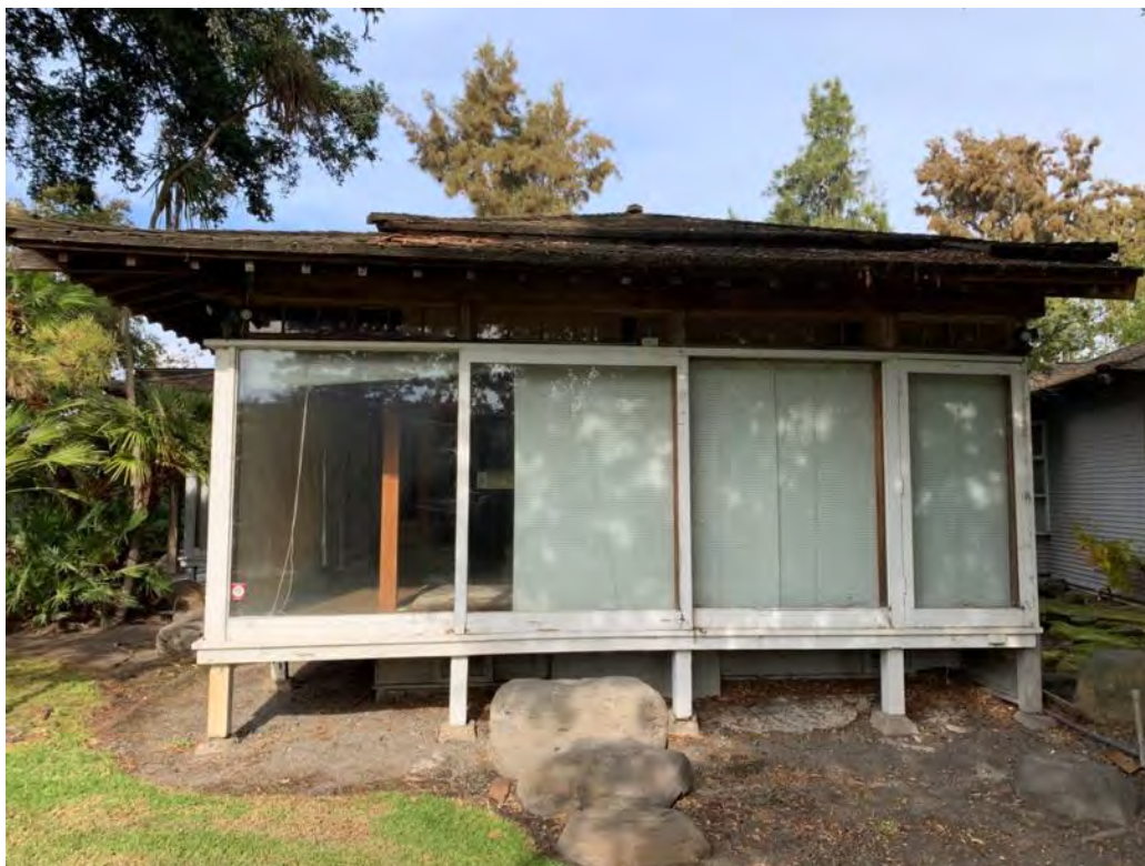
Tea house south elevation showing sliding glass doors with transoms and stepping stones
