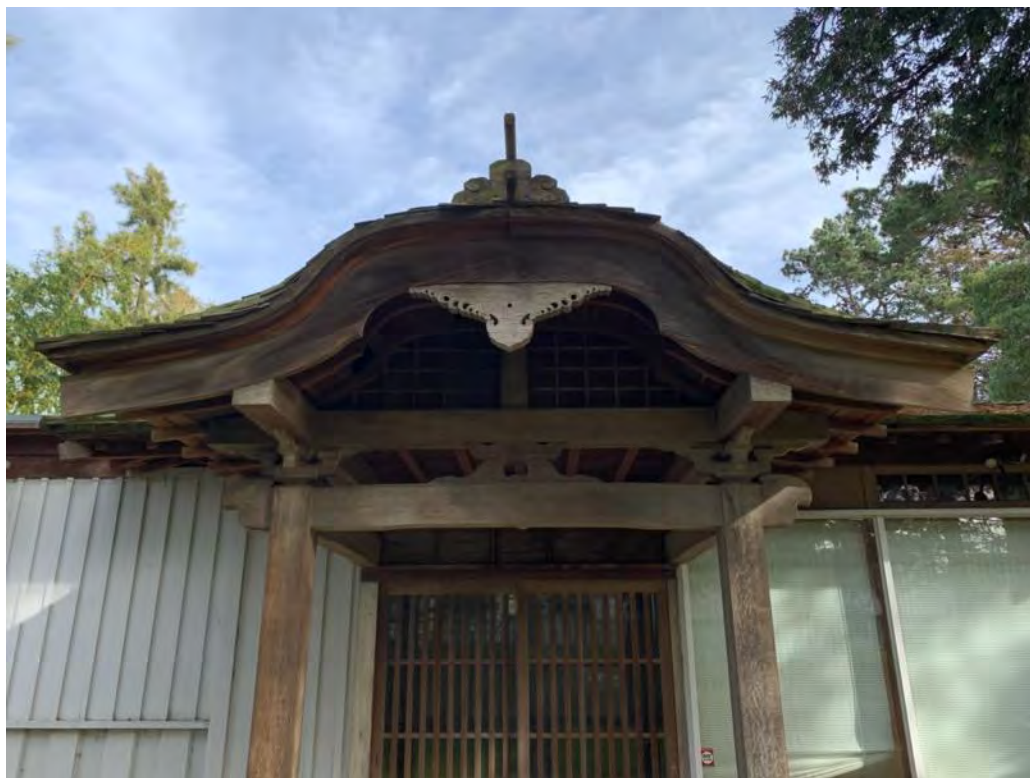
Tea house west elevation showing detail of kara-hafu style cusped gable roof
