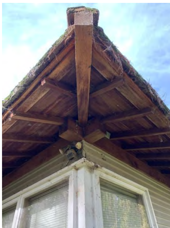
Southeast corner detail of tea house/residence showing flared roof eaves ( sumi-domo ), and exposed rafter tails at the corner intersection of the roof ( sumi-ga ).
