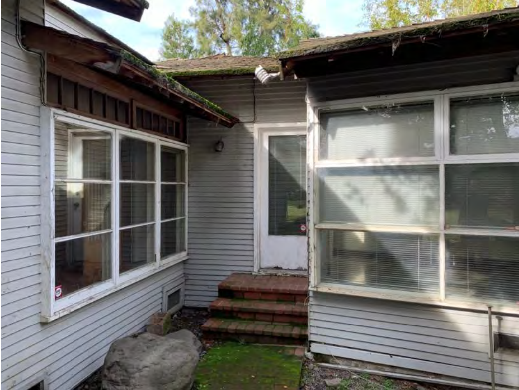
Tea house east and south elevations showing side door to kitchen and 'knuckle' attachment of residential addition
