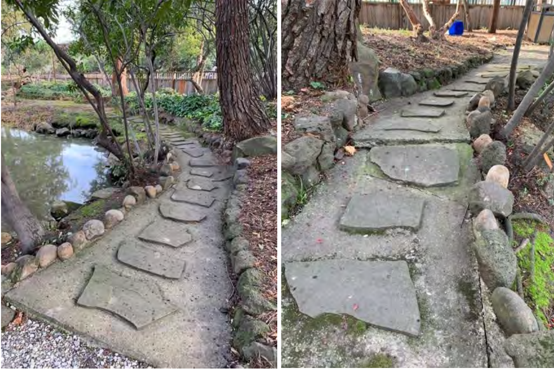
View of curvilinear stone and concrete path looking southeast (left) with cracked cement detail looking northwest (right)
