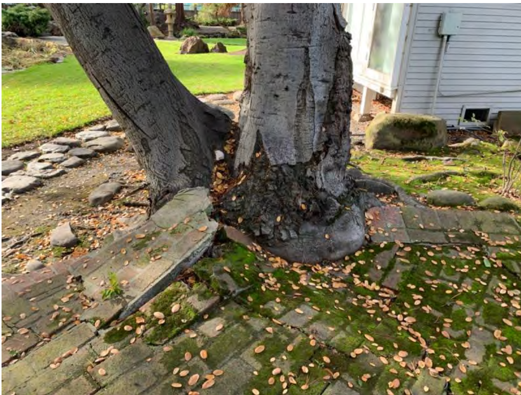
Southwest corner of brick patio disturbed by oak tree roots looking west
