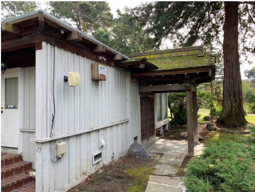
View of northwest corner of Tea house/residence showing primary entry on west elevation with its kara-hafu style cusped gable roof and supporting posts and beams
